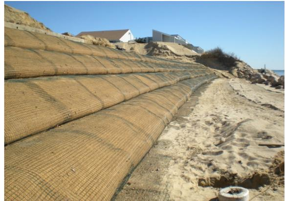
High energy wave impacts were a complicating factor at the site that factored into the design. Most soft solutions have been found effective in low impact sites, but the nature of this site demanded a more robust solution to withstand wave and debris forces at the site.
