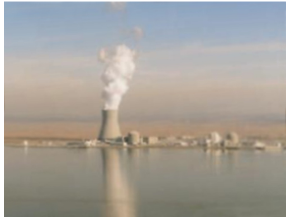
Salem Generating Station
