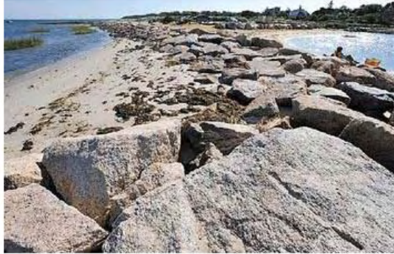
Brewster officials are weighing construction of a stone wall to slow the erosion that is threatening to wash away the parking lot at Paines Creek Beach.
